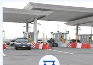
toll collection system
